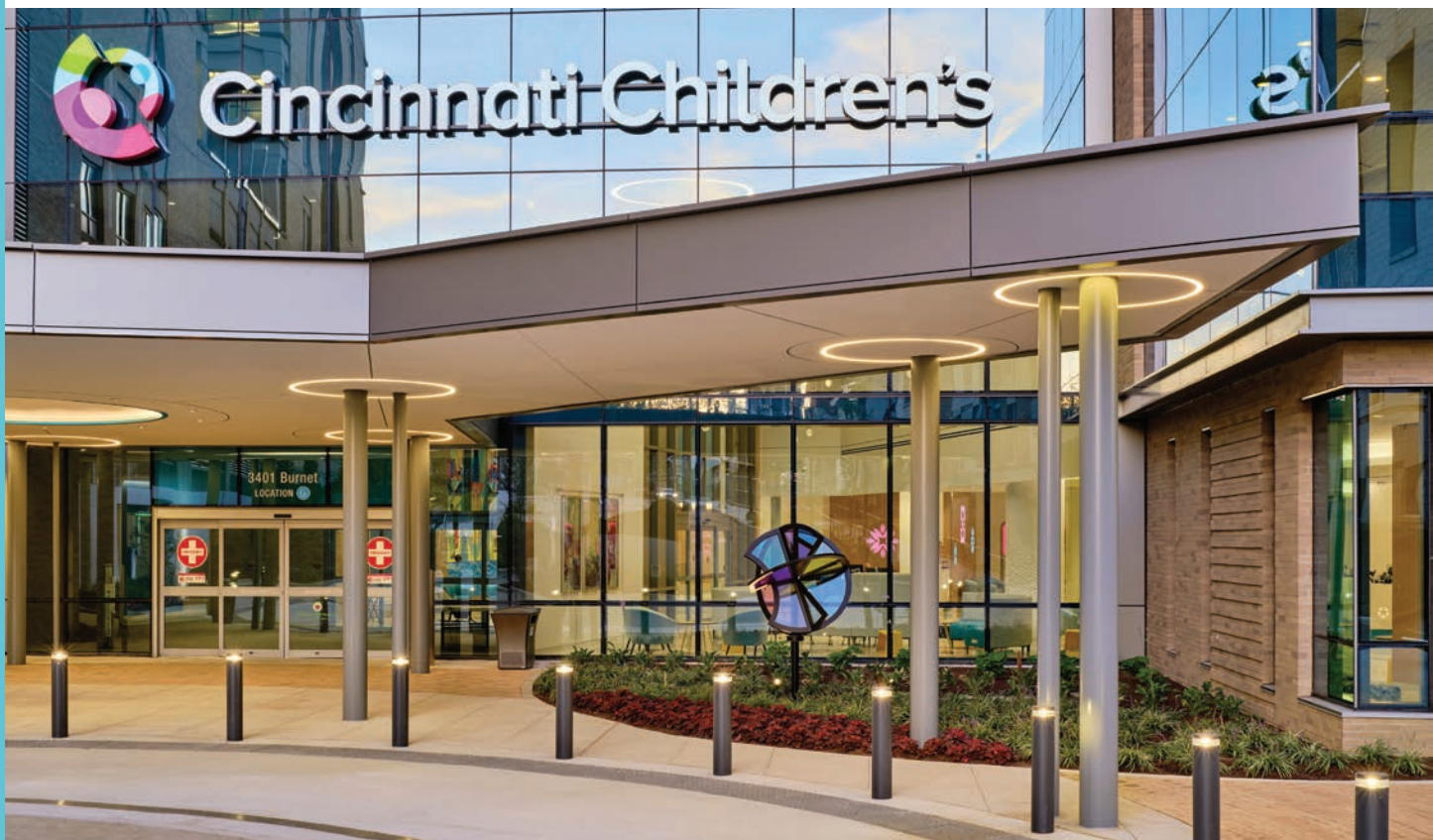
Cincinnati Children's Hospital Medical Center Photo courtesy of CCHMC
